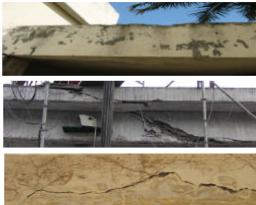
Fig. 7: Visual data of some damaged beams
