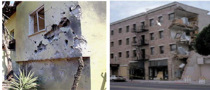
Fig. 2: Example of cases -Moderately damaged-MD
