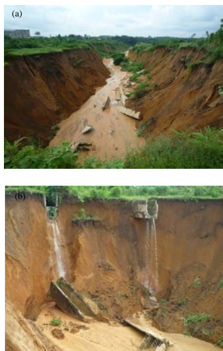
Fig. 5: a) Gully stretching towards the toe; b) An active gully that has damaged the drainage facilities
